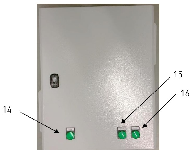
Figure 5: Front face of cabinet
